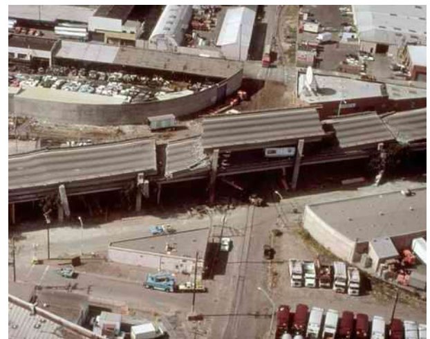
Figure 4. Road damaged by an earthquake ( www.recentearthquakes.net/resources/Earthquakes )
